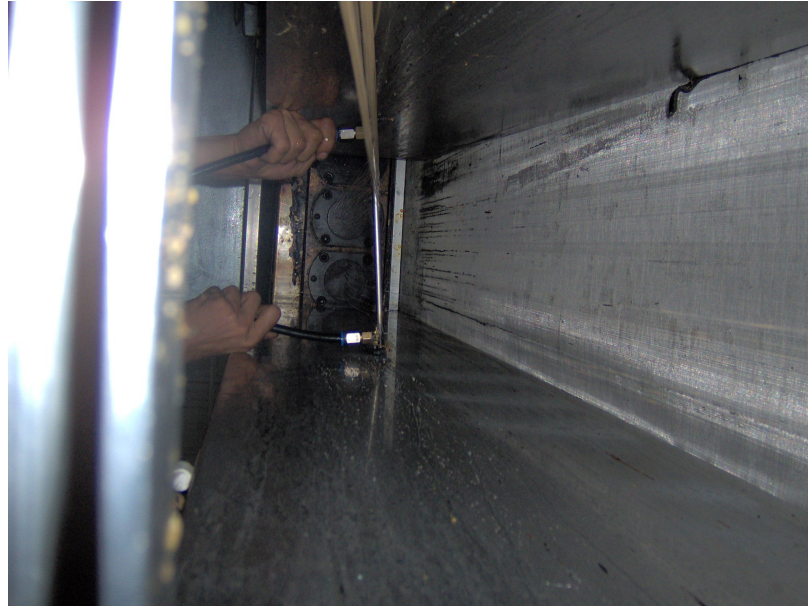
Figure 4.15 Adjusted the cooling pipe by hand.
