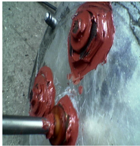
Photograph 2 : Sealing of cover
