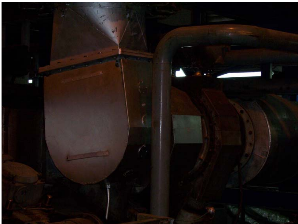
Figure 7.10 Front view of turbocharger NR34S in SANKO DEPC
