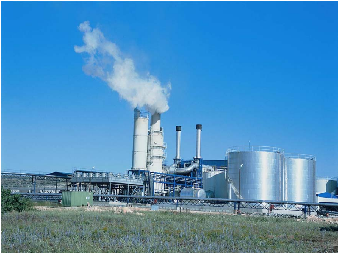
Figure 7.1 The plant overview of Sanko DEPC
