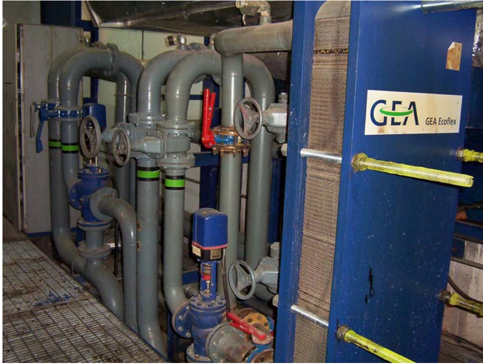
Figure 7.15 Intercooler (IC) in SANKO DEPC
