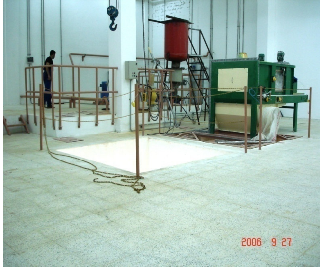
Figure 2.13 Liming Unit.
