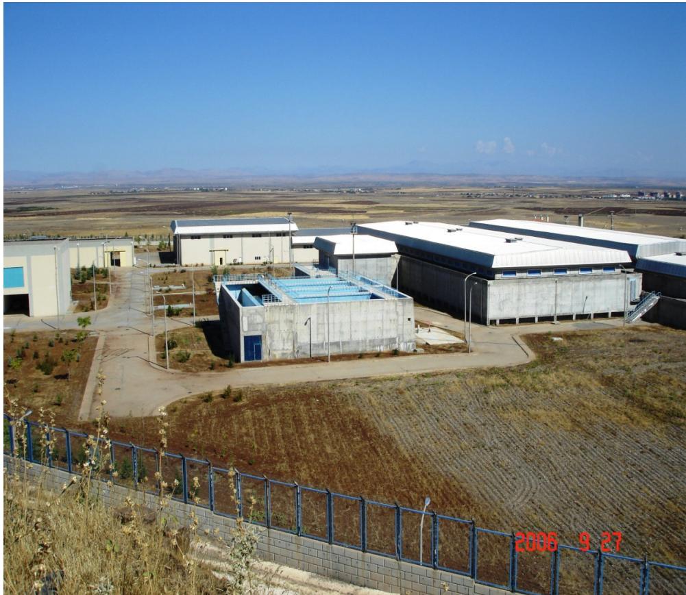
Figure 2.19 Diyarbakır Drinking Water Treatment Plant.
