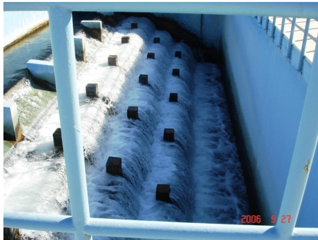
Figure 2.6 Aeration Structure.
