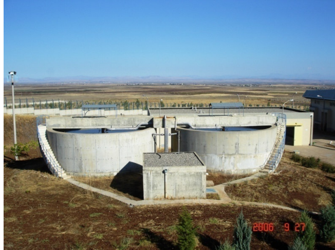
Figure 2.15 Sludge Digesters.
