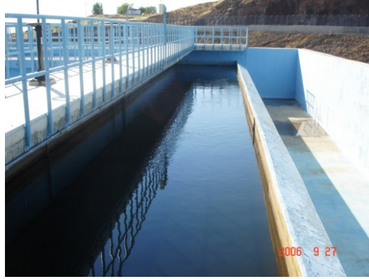
Figure 2.7 Aeration Tank.
