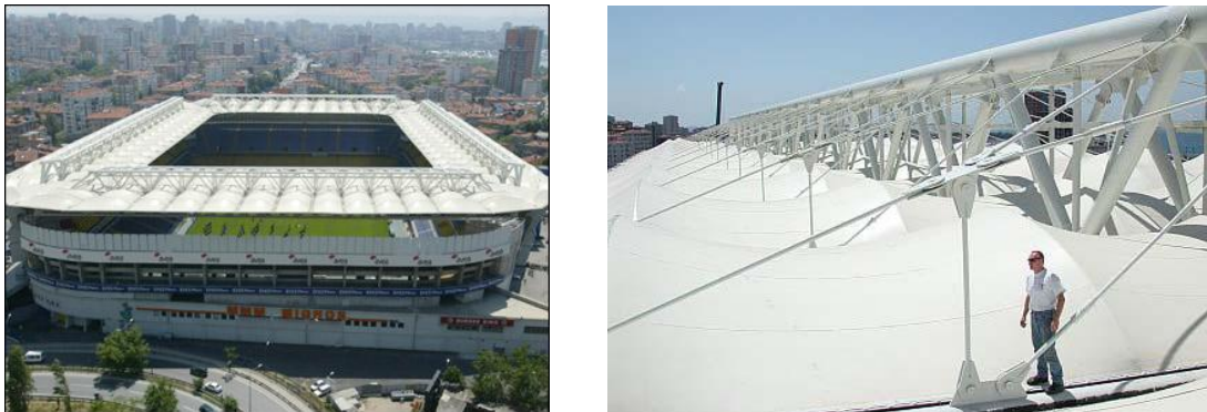
Figure 2.21 Stadium roofing for the Turkish soccer club Fenerbahce Istanbul
