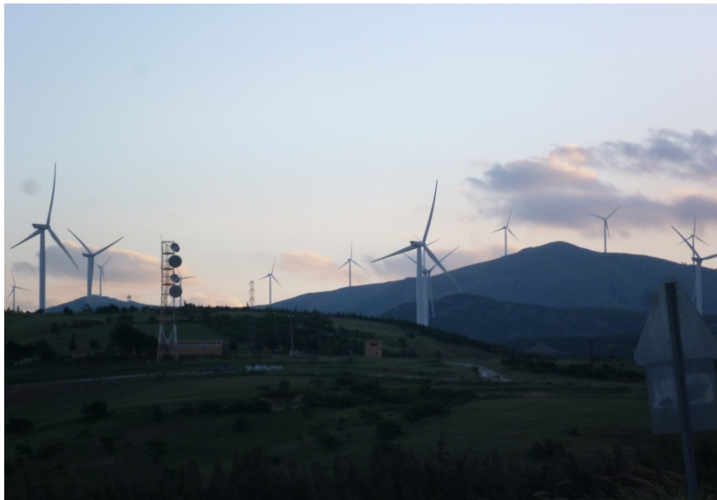
Figure 1. 2. Gökçedağ Wind Farm - Bahçe/Osmaniye - Turkey
