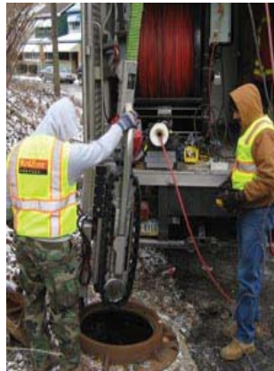
Figure 3.15 Large diameter pipe inspection systems [44].
