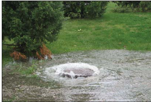
Figure 2.1 Water escapes through a manhole during an overflow event [6].
