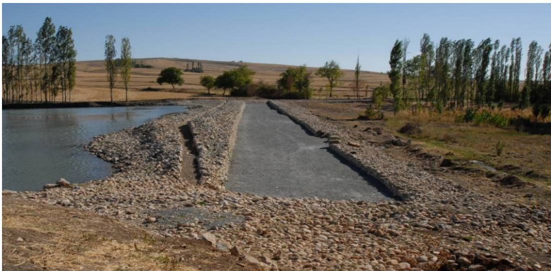
Figure 2-2 Hitit Dam- First dam in Anatolia
