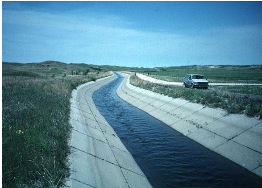
Figure 2.1. An Irrigation Open Channel (Canals and Navigable Rivers, 2012)
