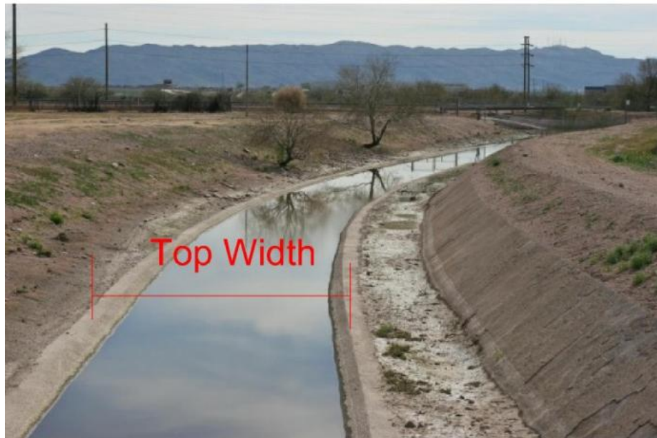
Figure 2.8. Top Width or Exposed Surface (StructureHUB, 2009).
