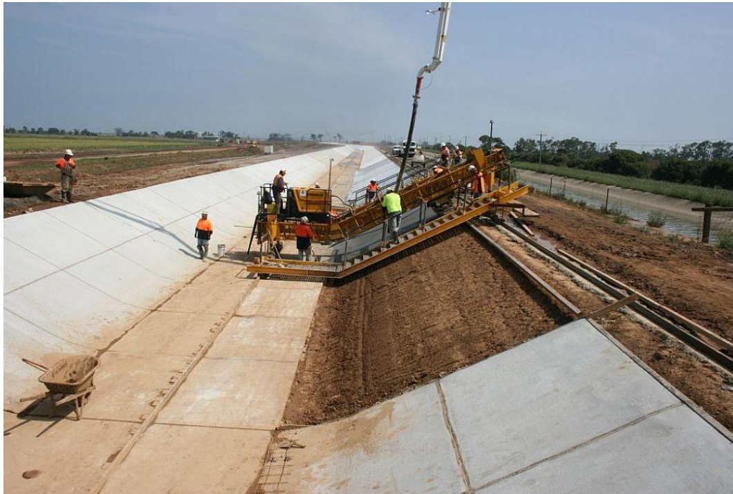
Figure 2.7. Lining Process in Open Channels (Worksafe awards, 2012).
