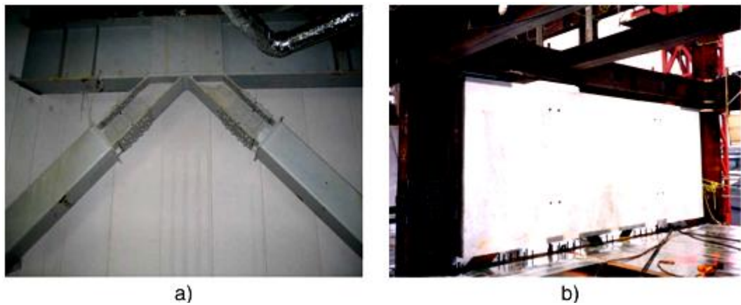
Figure 2.18 Photos of buckling-restrained braces a) typical tube BRB and b) panel BRB (Qiang, 2005)
