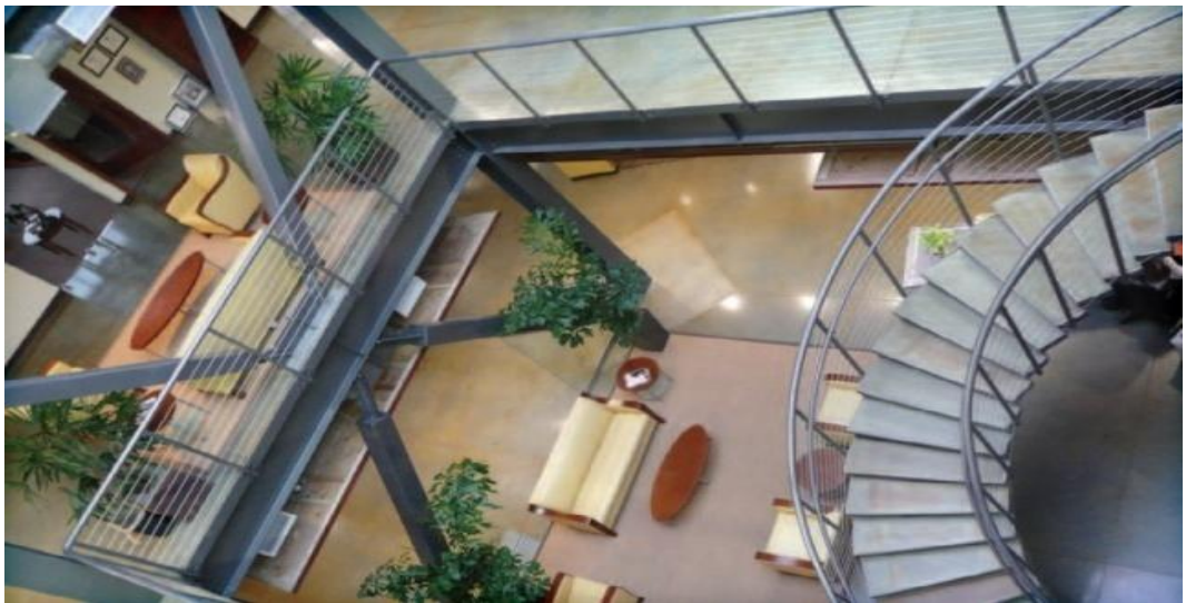
Figure 2.23 Use of BRB in SME steel corporate headquarter, West Jordan, Utah. (Corebrace, 2002)
