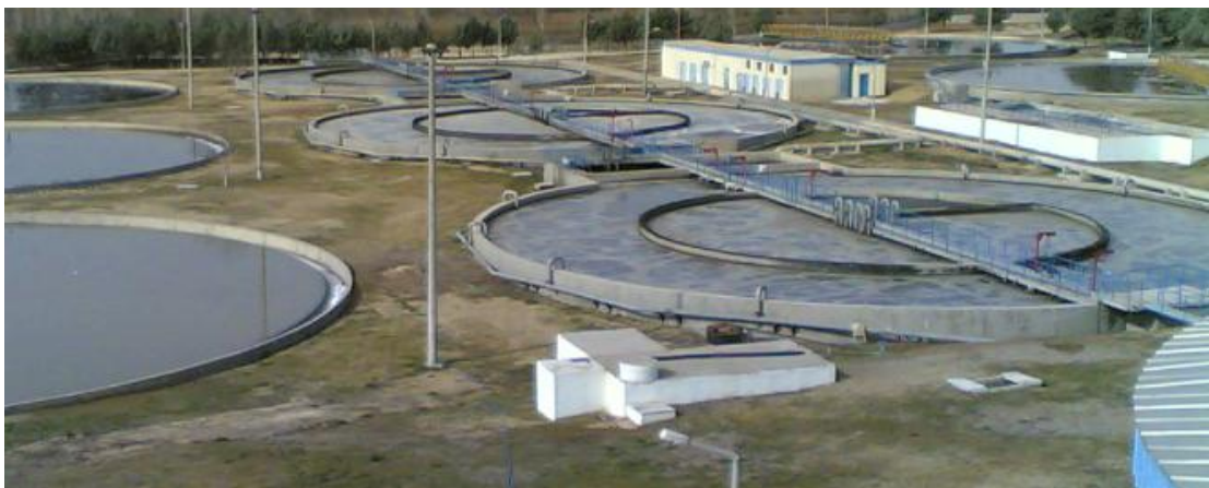
Figure 7.5: Aeration tanks of the GASKI WWTP
