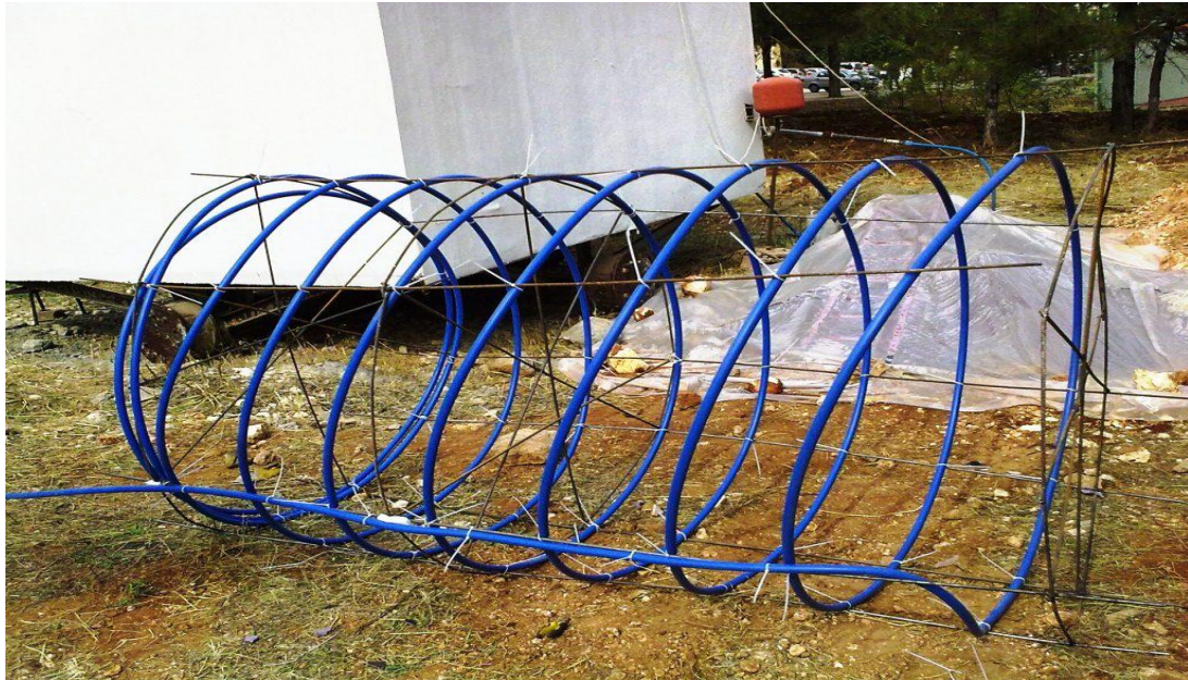
Figure 4.4. Slinky type ground heat exchanger before burying
