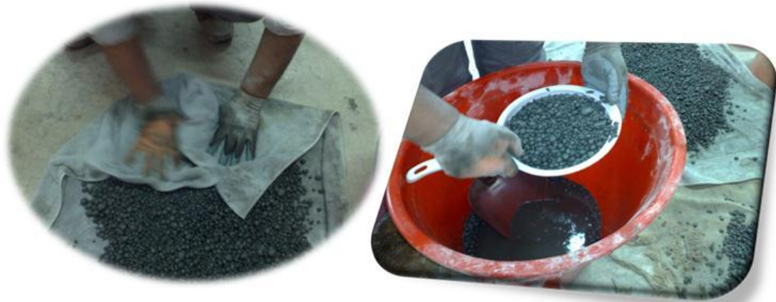
Figure A.5 Lightweight aggregate immersed in water before mix to get saturated surface dry aggregate aggregate
