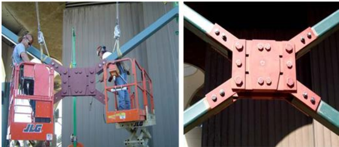
Figure 2.31 Pall friction damper in cross bracing (Shao et al., 2006)
