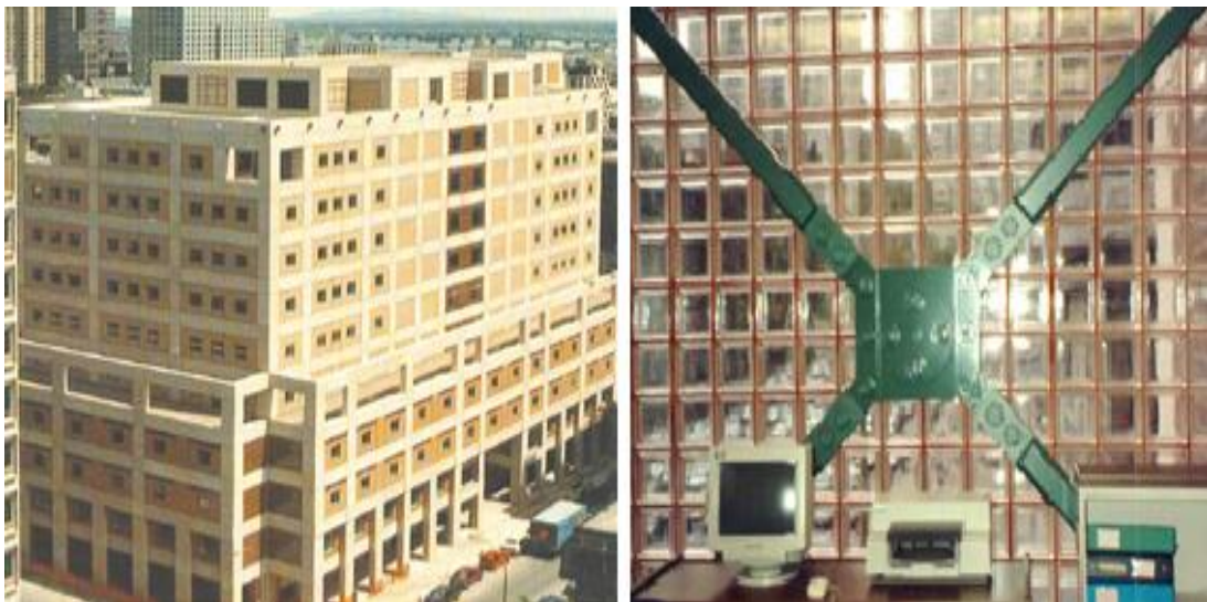
Figure 2.27 View of a) Concordia library building and b) Pall friction damper in cross bracing (Pall and Pall, 2004)
