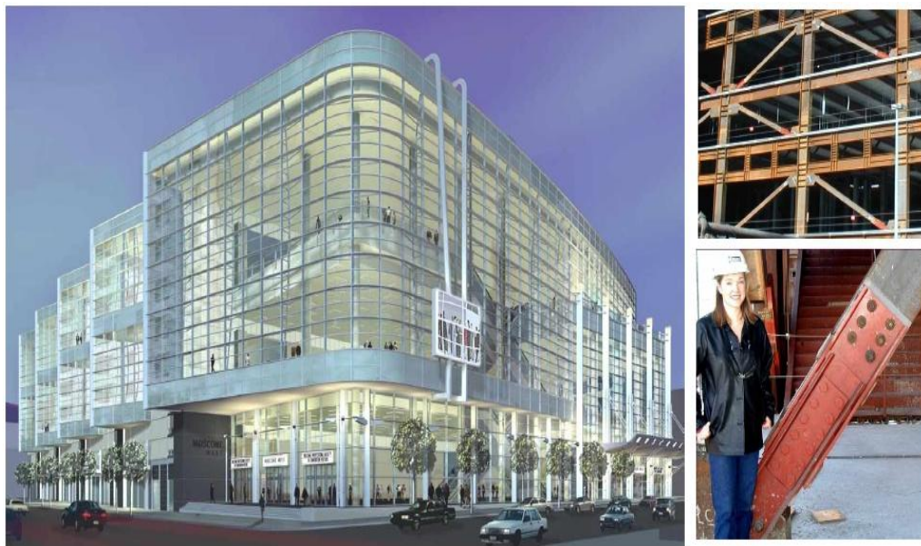
Figure 2.23 a) View of Moscone West convention center, USA and b) Pall friction dampers (Pall and Pall, 2004)
