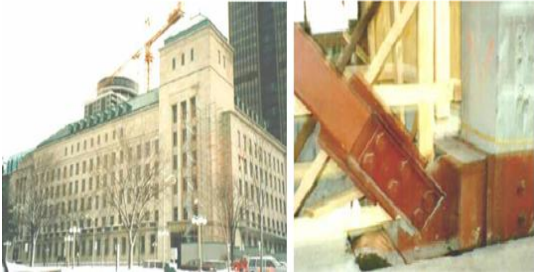
Figure 2.28 View of a) Justice headquarters and b) Pall friction damper (Pall and Pall, 2004)
