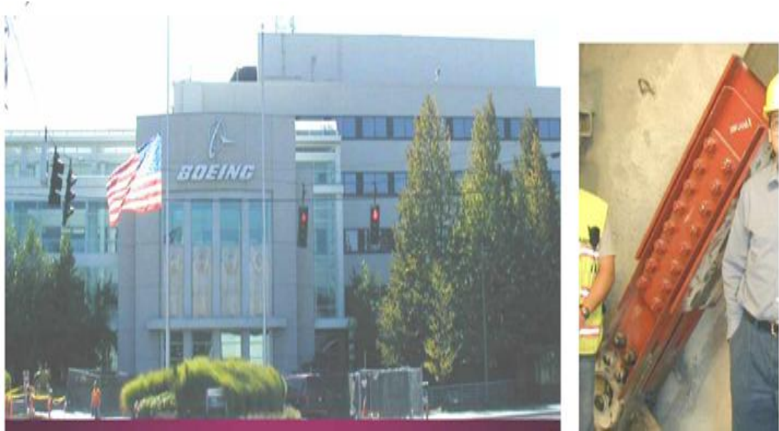
Figure 2.24 a) View of Cafeteria, Auditorium, and fitness building and b) Pall friction dampers (Pall and Pall, 2004)
