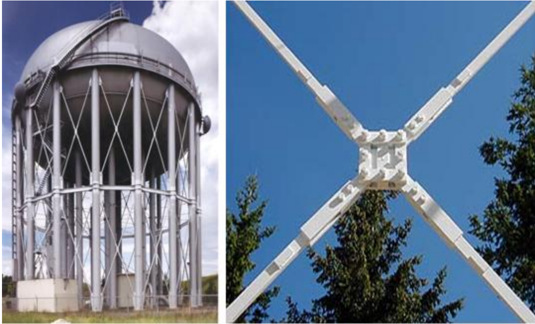
Figure 2.26 View of a) Million Gallon reservoir water tank and b) Pall friction damper (Pall and Pall, 2004)
