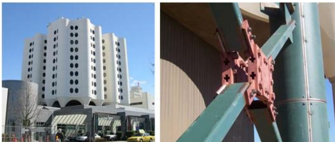
Figure 2.29 View of St. Joseph medical center patient tower with friction damper (Shao et al., 2006)
