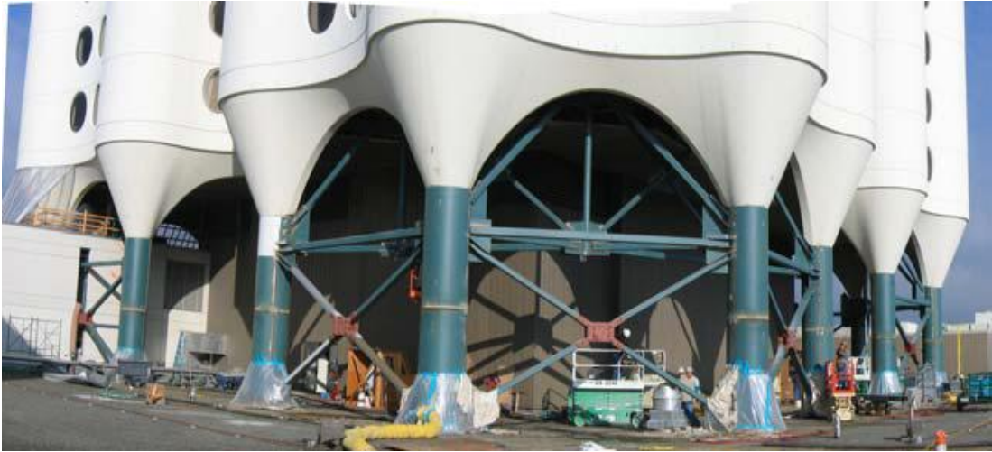
Figure 2.30 Seismic upgrade with cross-brace friction dampers (Shao et al., 2006)
