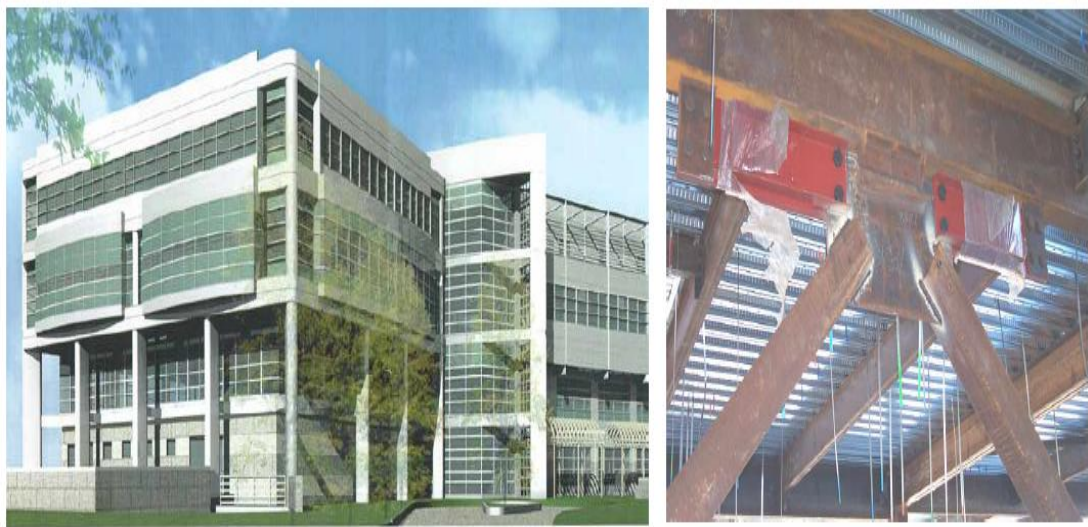
Figure 2.25 a) View of Ambulatory care center and b) Pall friction dampers (Pall and Pall, 2004)
