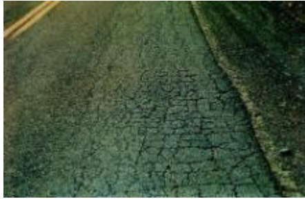
Fatigue cracking
