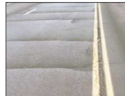
Figure 2.3 Reflective cracking (Miller and Bellinger, 2003)
