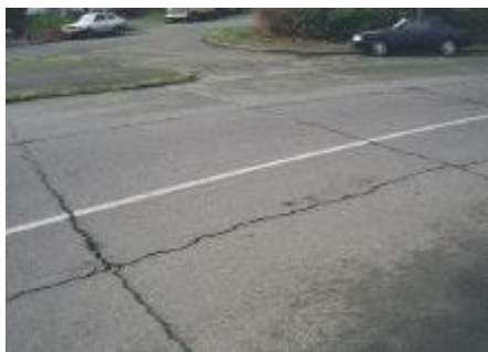
Figure 2.3 Reflective cracking (Miller and Bellinger, 2003)
