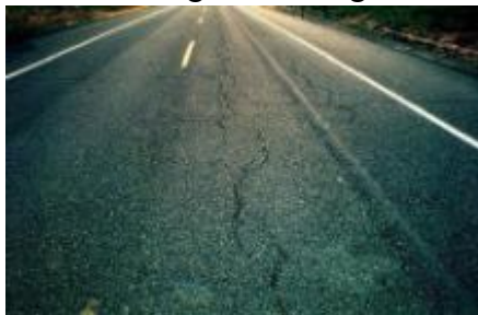
Logitudinal cracking
