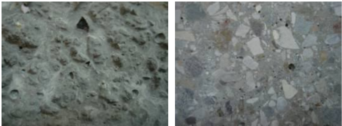
Figure 3.33 Typical close-up view of untreated rough and smooth concrete surfaces
