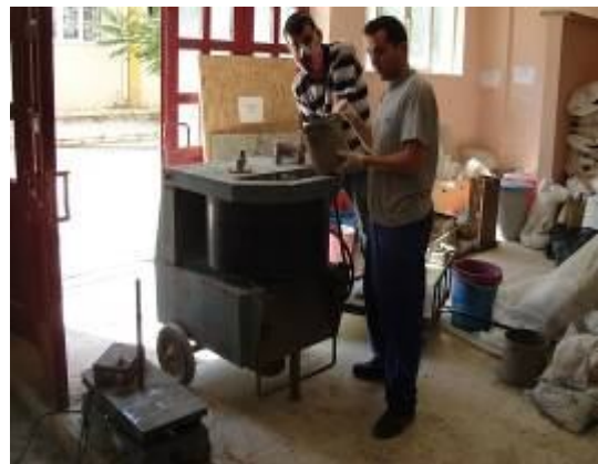
Final mixing of all materials
