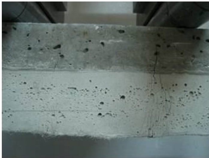
b) S_ECC composite beam after four point bending test
