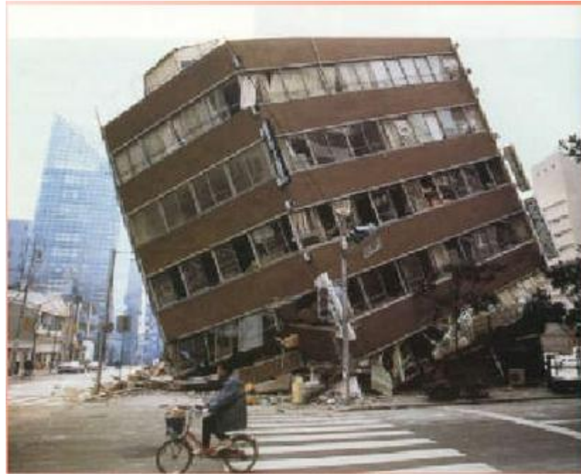
Figure 2.2 Scenes of damaged structures, Kobe (Japan) 1995 ( www.slideshare.net/IBGeogIST/2004-indian-ocean-tsunami-2109248 )
