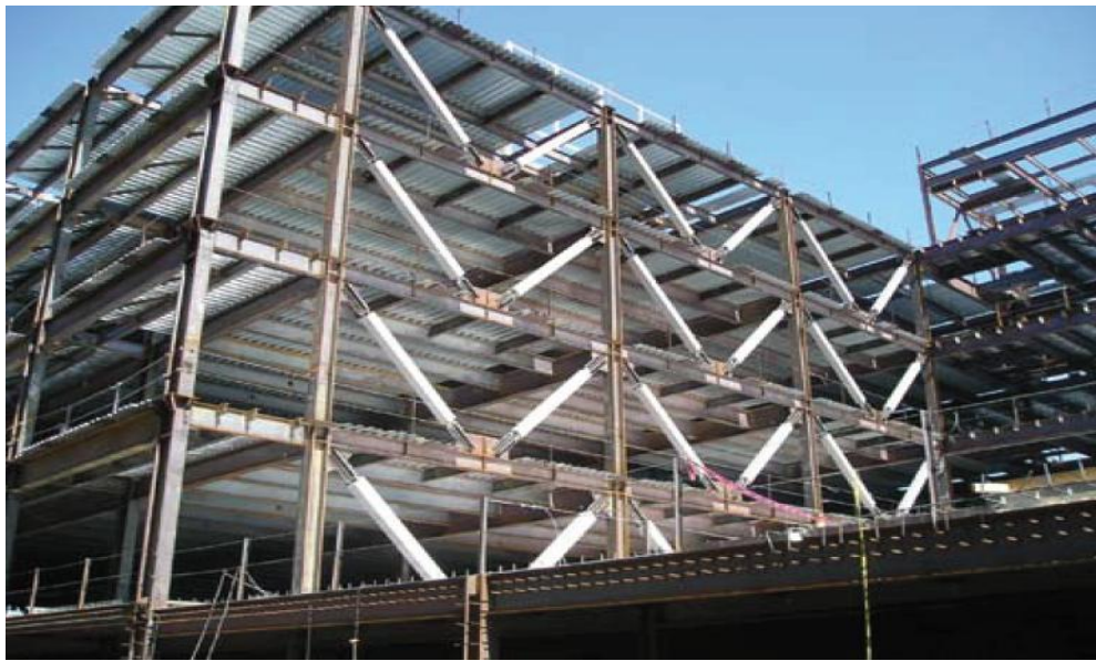
Figure 2.35 Application of BRBs (Walterio and López, 2008)
