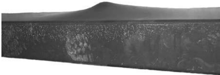
Figure 2.8 Bulging of steel casing (courtesy of Star Seismic, LLC) (Uang and Nakashima, 2004)
