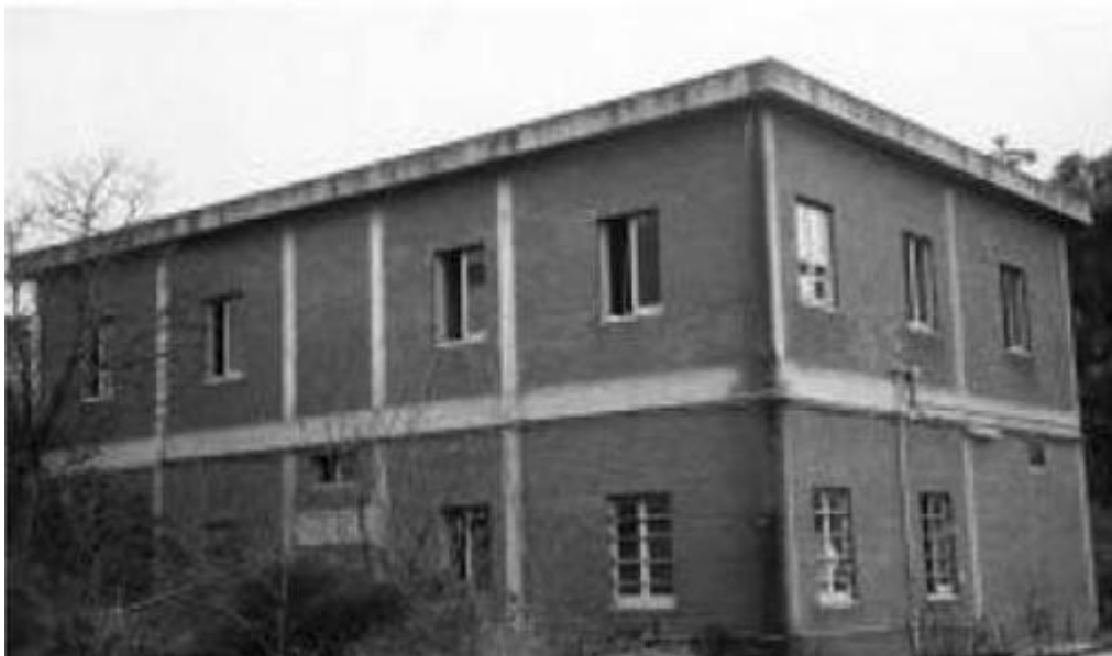
Figure 2.32 The tested reinforced concrete structure in its original condition (Bagnoli Naples, Italy) (D'Aniello et al., 2009)
