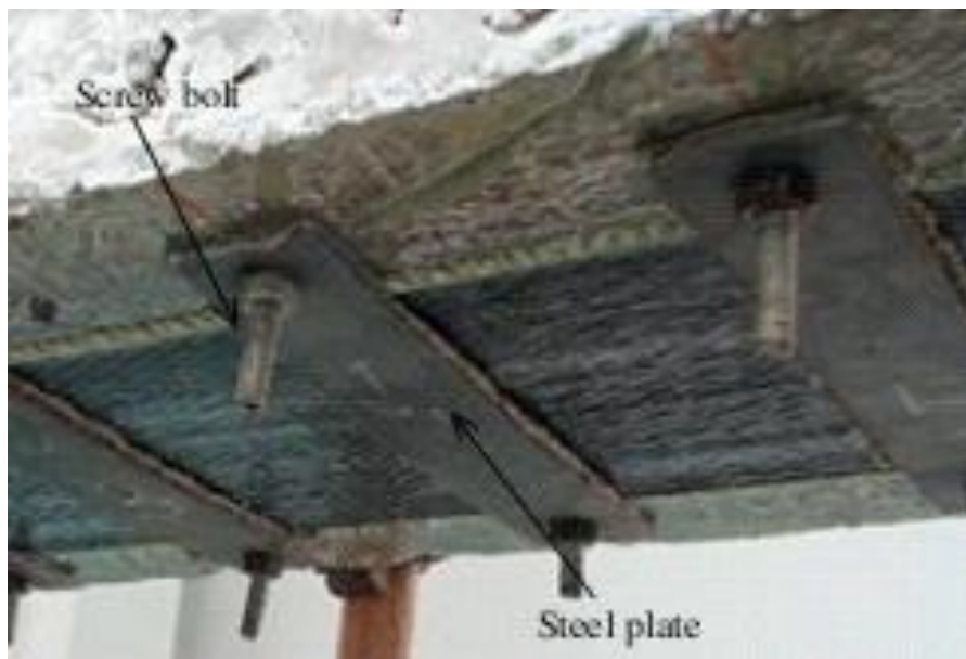
Figure 2.5 Pin mechanical fastened technique (Zhou et al., 2012)
