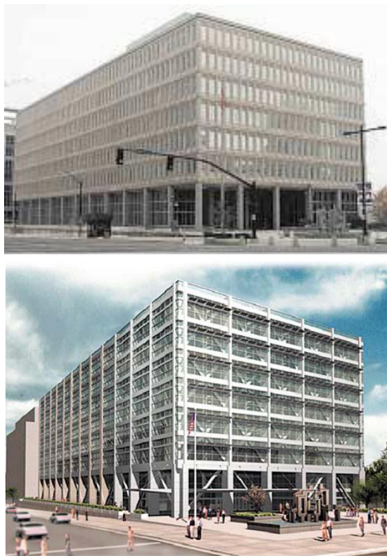
Figure 2.26 Wallace F. Bennett Federal building (Brown et al., 2001)
