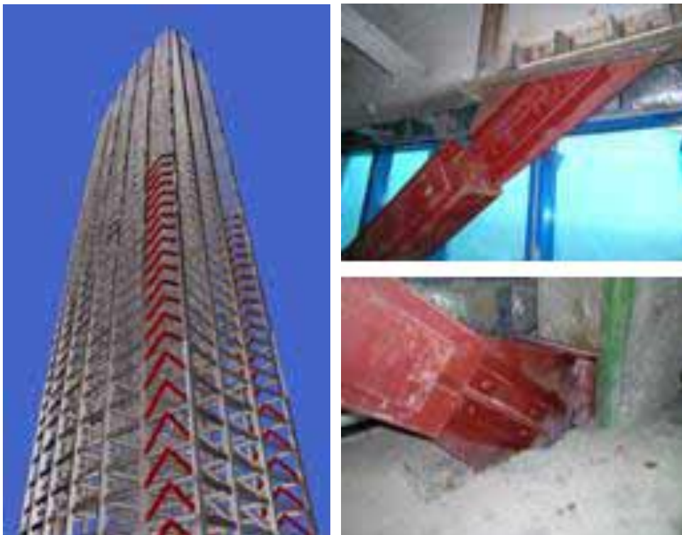
Figure 2.24 The 3D model of Shee-Hwa United World Tower and BRB details (in Taichung) (Tsai et al., 2004)
