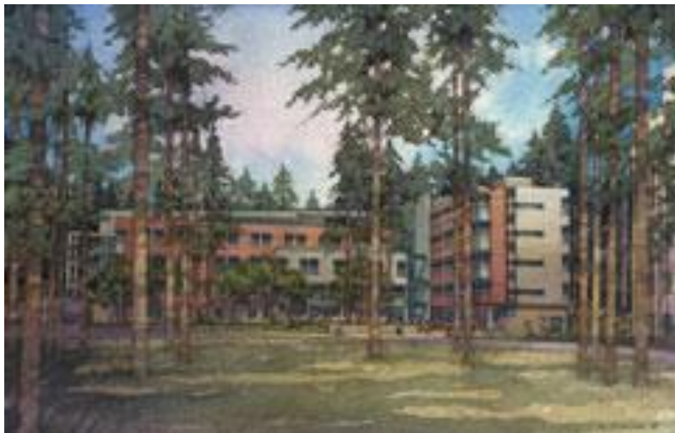
Figure 2.18 Physical sciences building in University of California at Santa Cruz, California (PEER, 2002)
