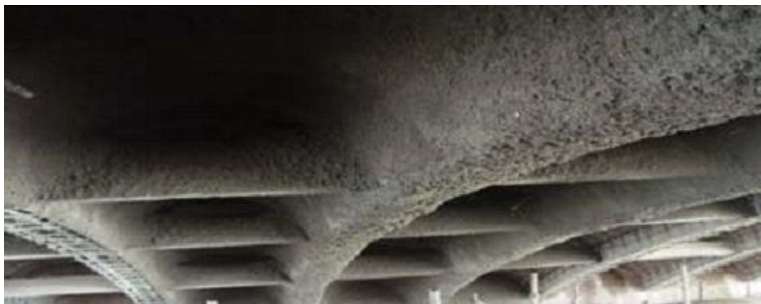
Figure 2.4 The first layer of sprayed concrete (Naser and Zonglin, 2011)
