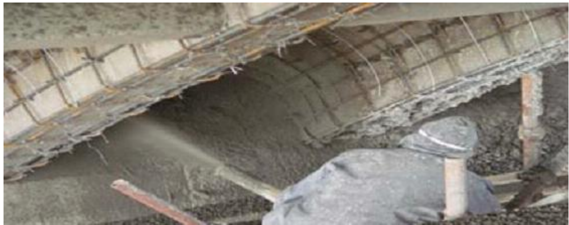
Figure 2.3 Spraying the concrete (Naser and Zonglin, 2011)
