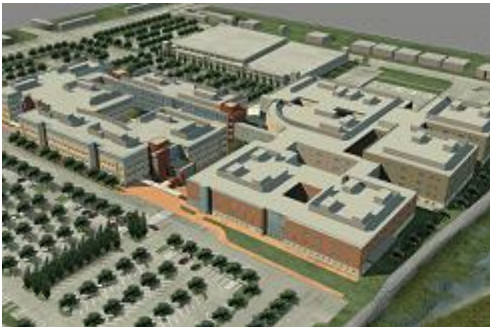
Figure 2.20 Kaiser Santa Clara medical center hospital building: Phase I, Kaiser Permanente, Santa Clara, California (PEER, 2002)
