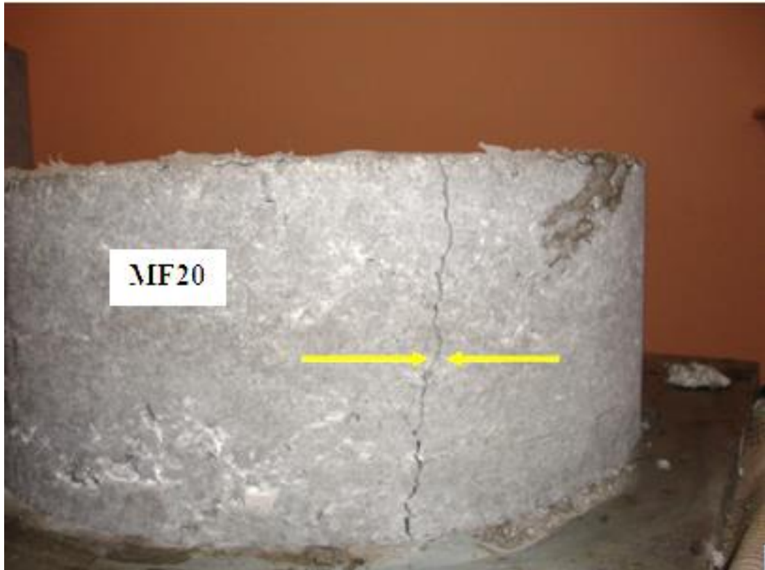
Figure 3.16 Photographic view of a cracked ring specimen (MF20)
