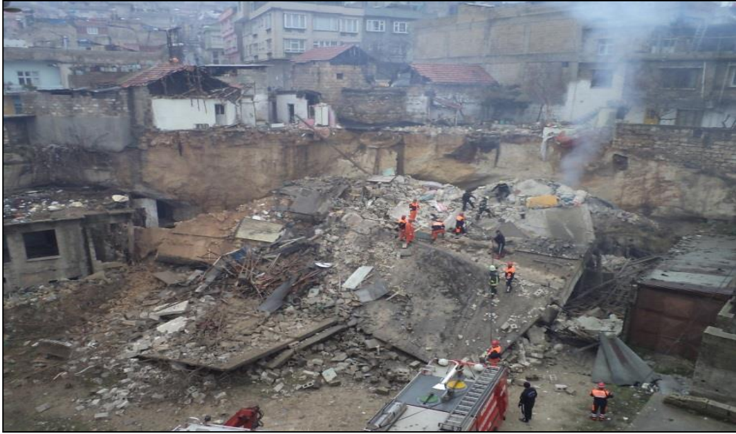
Figure 1.1 View of the partially collapsed cave named Üzümcü in Delbes Neighbourhood (Gaziantep Metropolitan Municipality)
