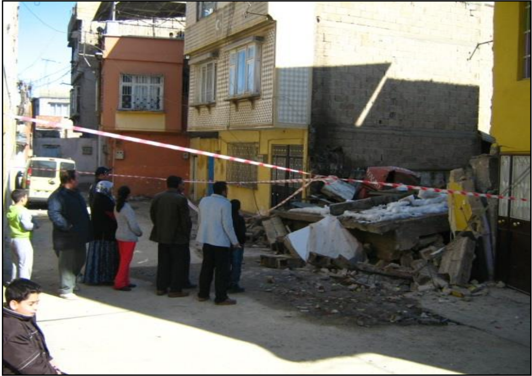
Figure 1.4 Appearance of the collapsed cave in Kılınçoğlu Neighbourhood
