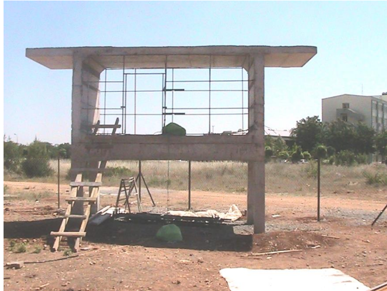
Figure 3.3 The box girder segment and the after formwork removal
