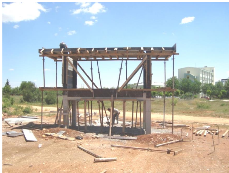
Figure 3.2 The formwork of the experimental box-girder segment
