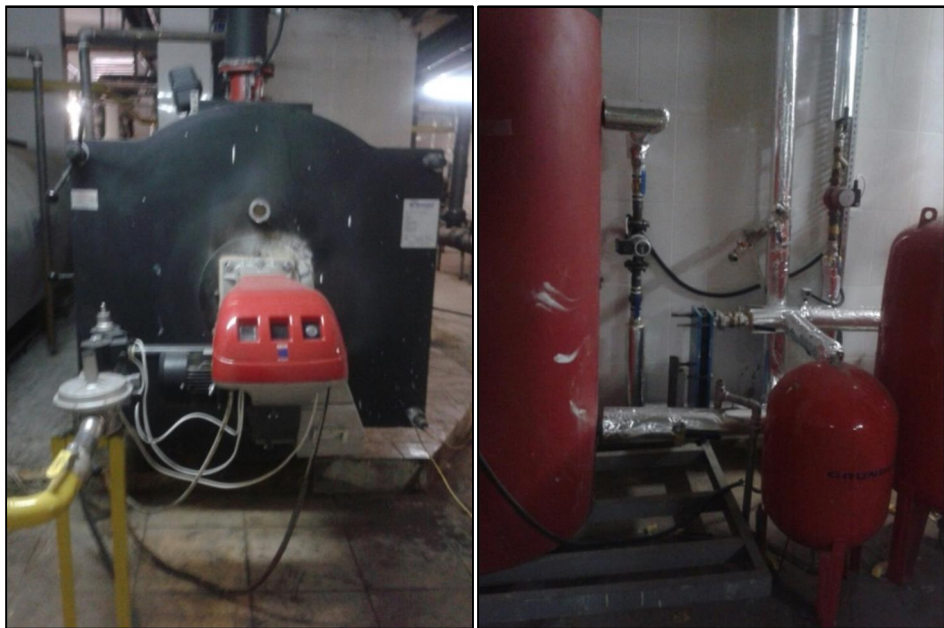
Figure 3.15 Boiler and heat exchanger zone line
