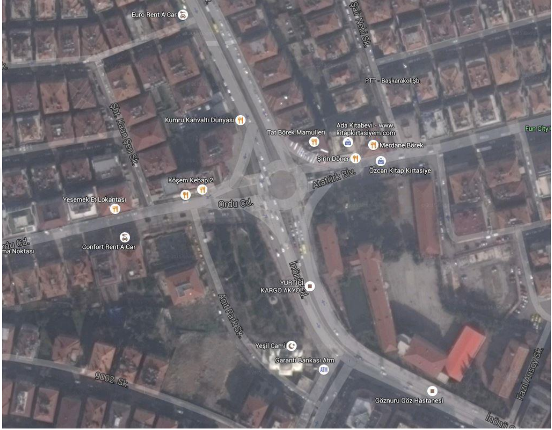
Figure 5.8 İnönü Avenue – Ordu Avenue Intersection
