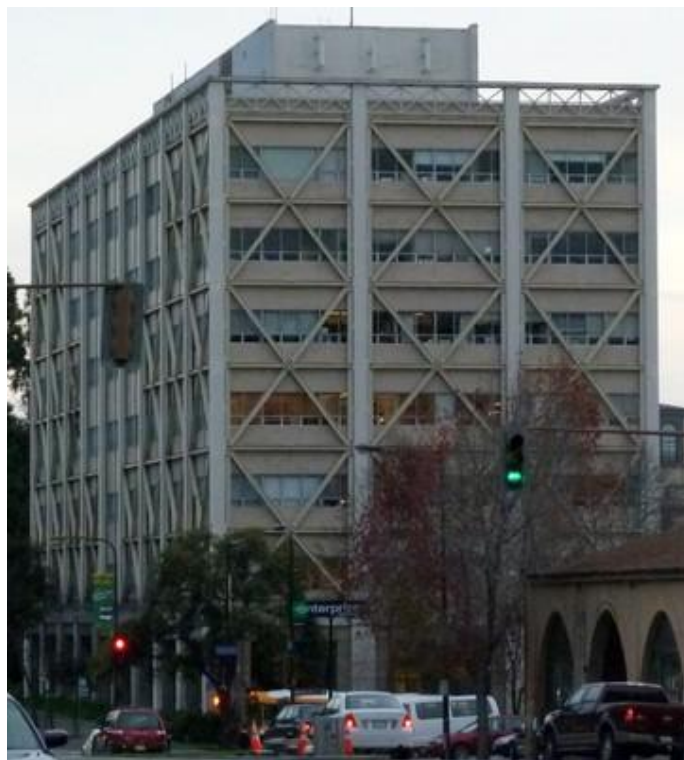
Figure 2.11 Exterior steel braced as a retrofit solution (Viswanath and Desai, 2008)
