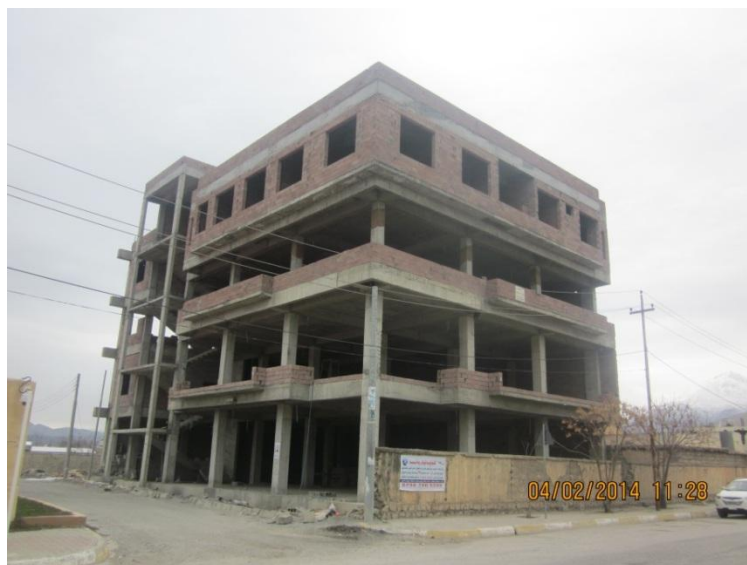
Figure 2.1 Residential Reinforced Concrete building in Soran, Erbeel
