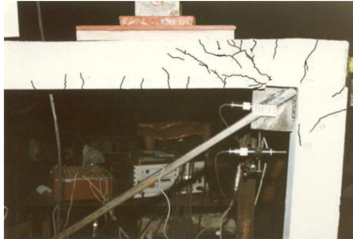
Figure 2.12 Increasing the stiffness of beam–column connection due to steel angle and gusset plate (Massumi and Absalan, 2013)
