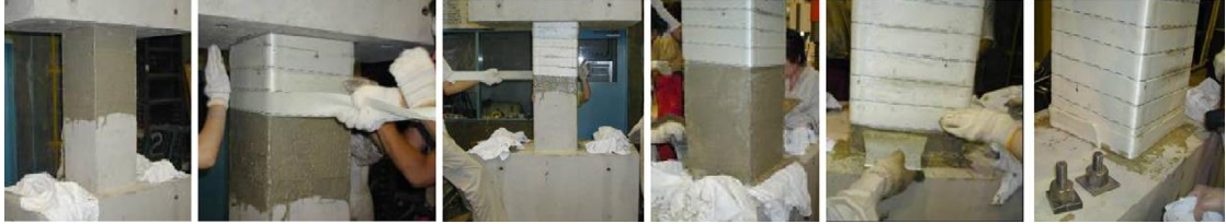
Figure 2.17 Column reinforcing process (Kim et al., 2012)
