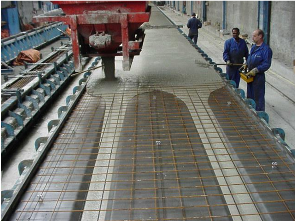
Figure 2.1 Casting precast element of SCC (EFNARC, 2005)
