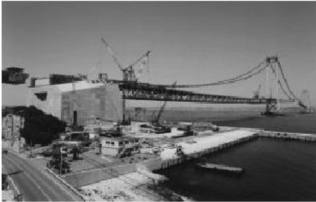
Figure 2.2 Akashi-Kaikyo Bridge, Japan (Ouchi and Hibino, 2000).
