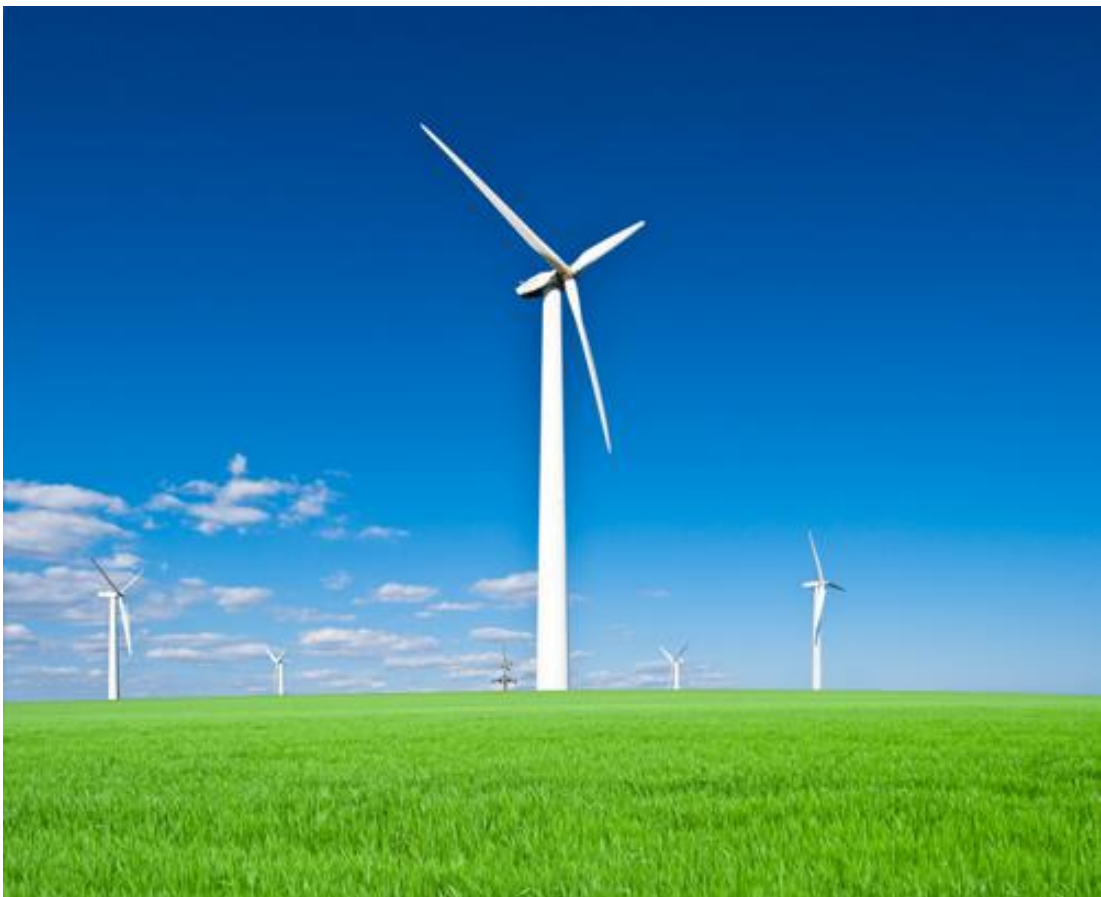
Figure 1.2 Wind Turbine in Power Plants [5]
