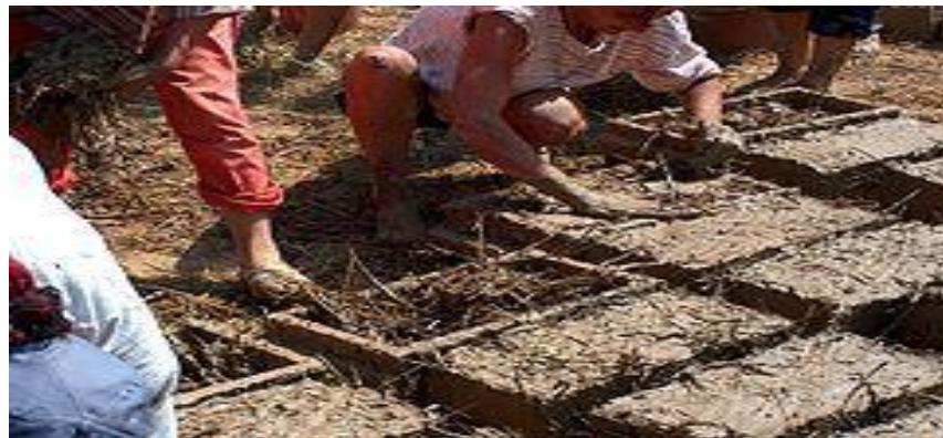
Figure 3.4 : Straw mixture of clay in the mud [15]
