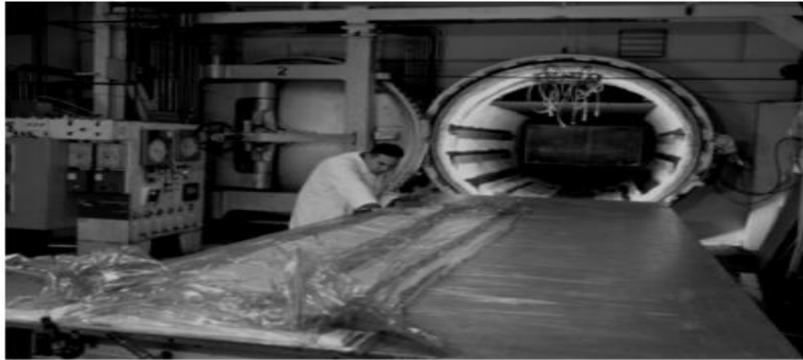
Figure 3.20 : A vacuum bagged composite aircraft part ready to enter the Autoclave [26]
