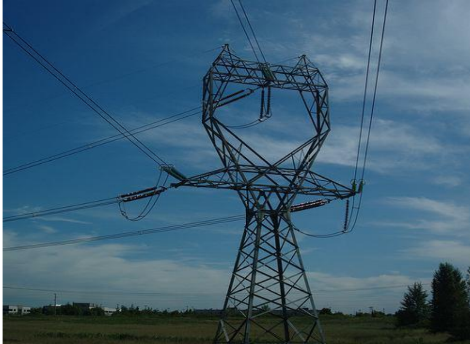
Figure 1.5 Single circuit - double lark or teal conductor.
