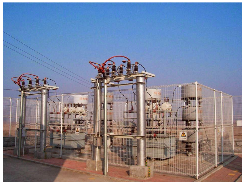
Figure 3.1. Single line diagram and practical shunt capacitor banks
