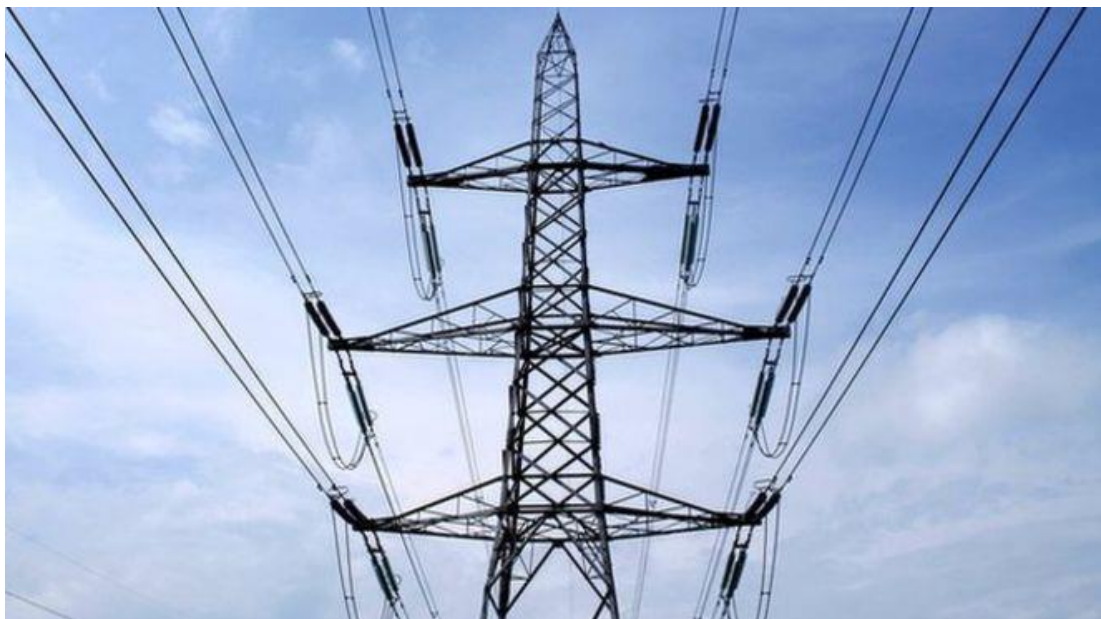
Figure 1.6 Double circuit - twin teal or lark conductor
