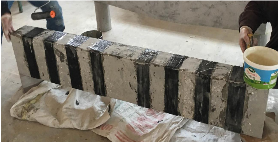
Figure 3.14 Using of knife and plastic roller to press the CFRP
