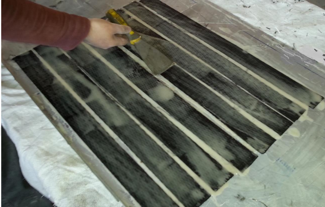
Figure 3.13 Process of impregnation of CFRP sheet with epoxy before installation.
