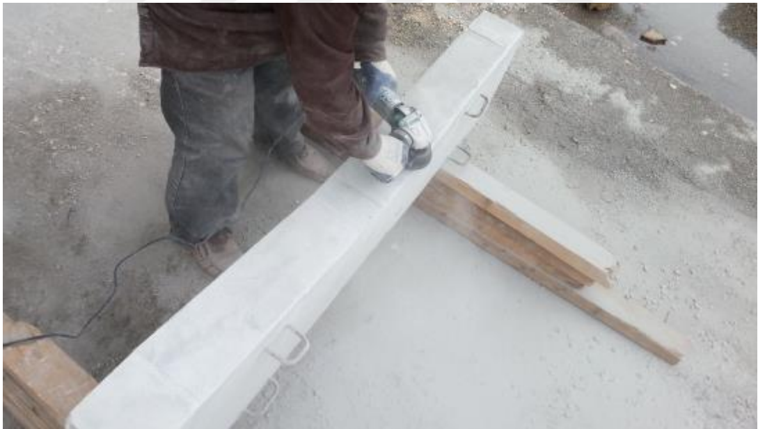
Figure 3.9 Grinding concrete surface before applying CFRP strips.
