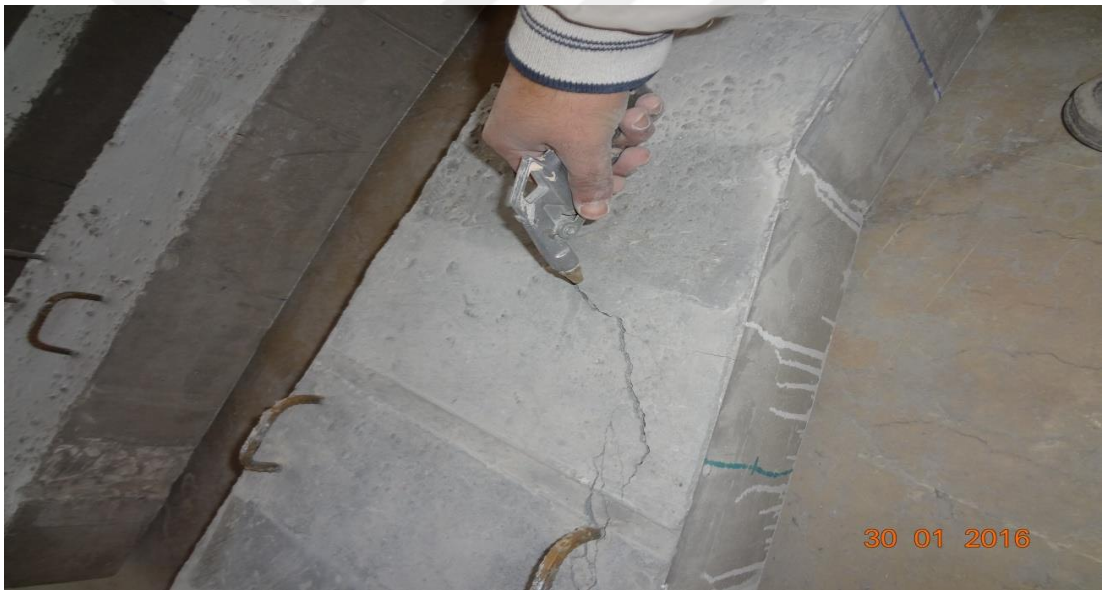
Figure 3.6 Cleaning of cracks by using compressed air.
