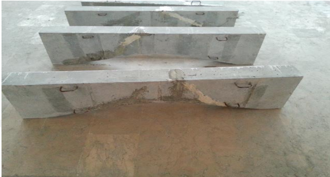
Figure 3.7 Sealing cracks of three faces of the beam
