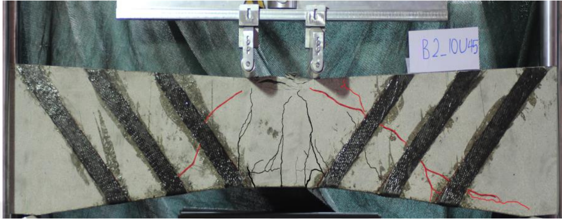
Figure 4.11 Failure mode of B2-10U45 beam
