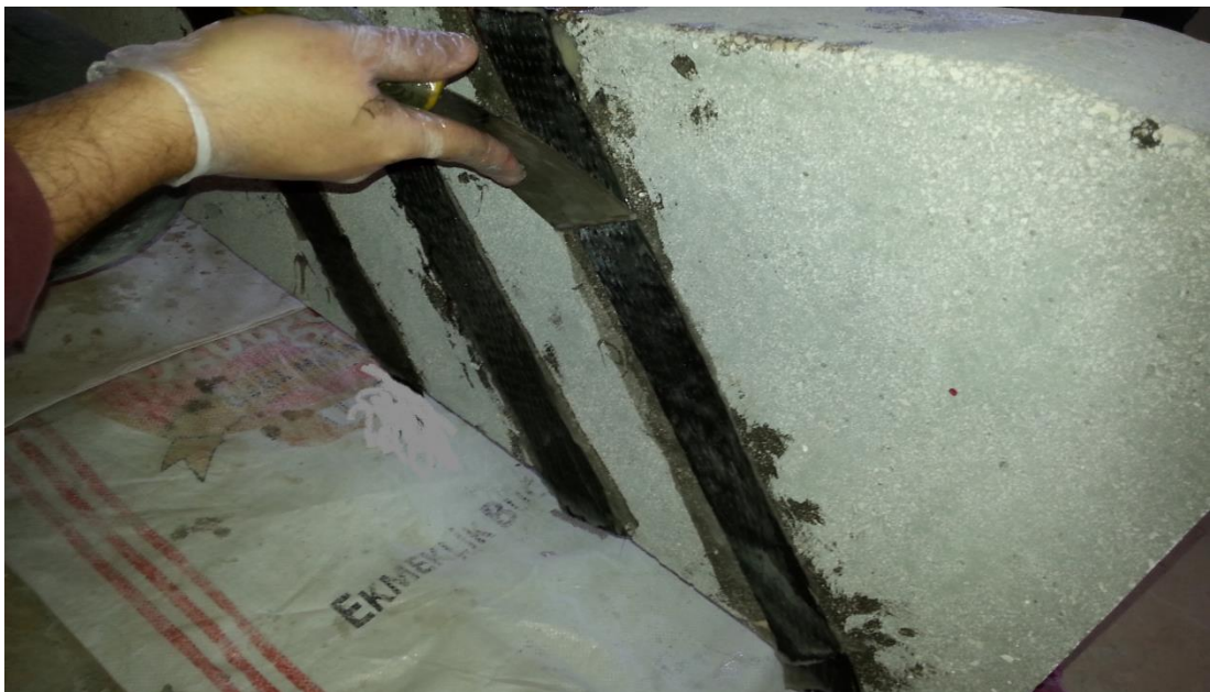
Figure 3.15 Method of compressing the CFRP using a knife.
