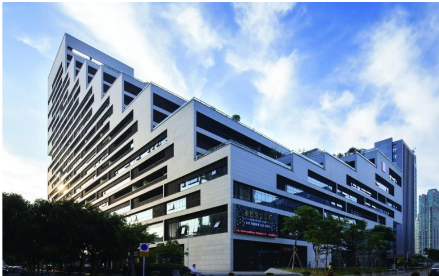
Figure 1.2 Shenye TaiRan Building in China 2012 ( www.archdaily.com )
