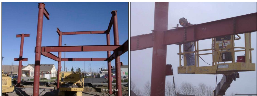
(c) Shop-fabricated CFT joint
