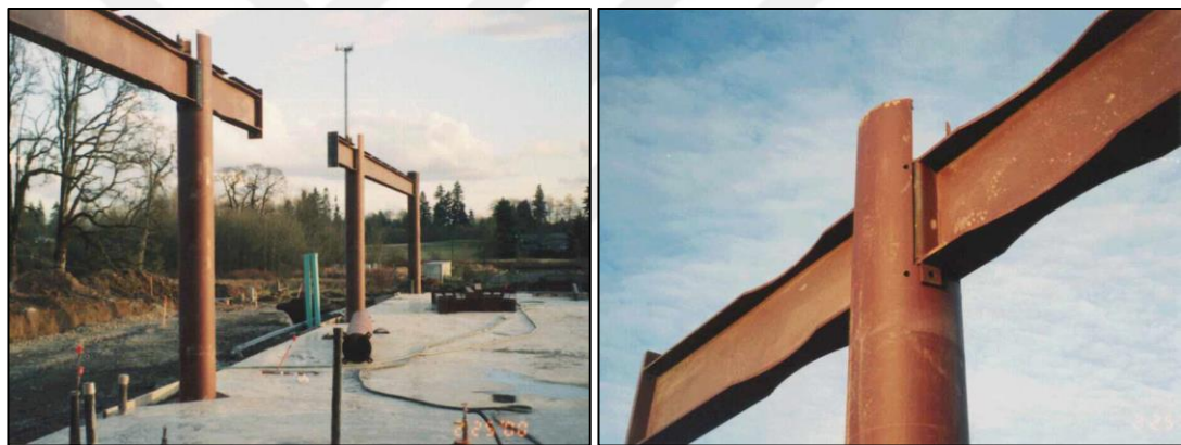
(a) Field-fabricated CFT joint
