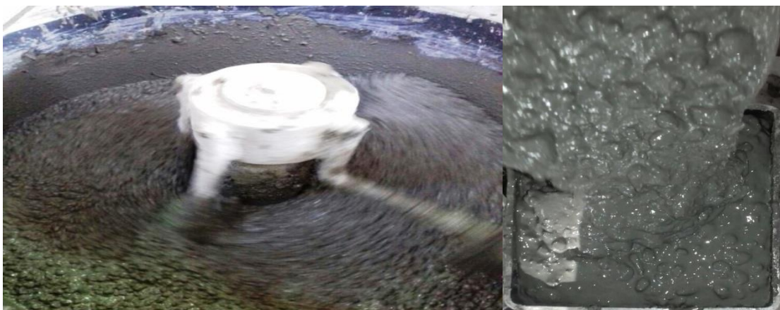
Figure 4.2 Final stages for lightweight concrete mixture
