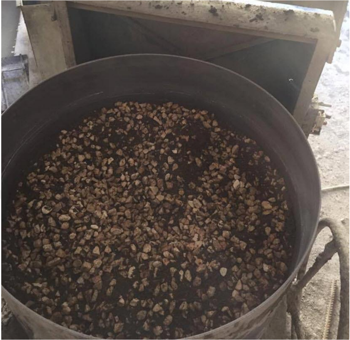
Figure 3.3 Photographic view of Mixing of concrete
