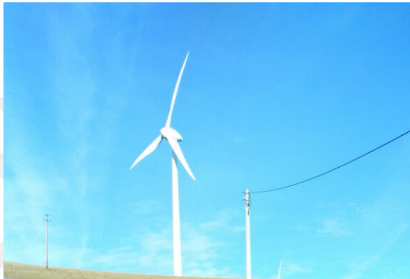
Figure 5. 2 A private wind turbine in Freiburg/Germany
