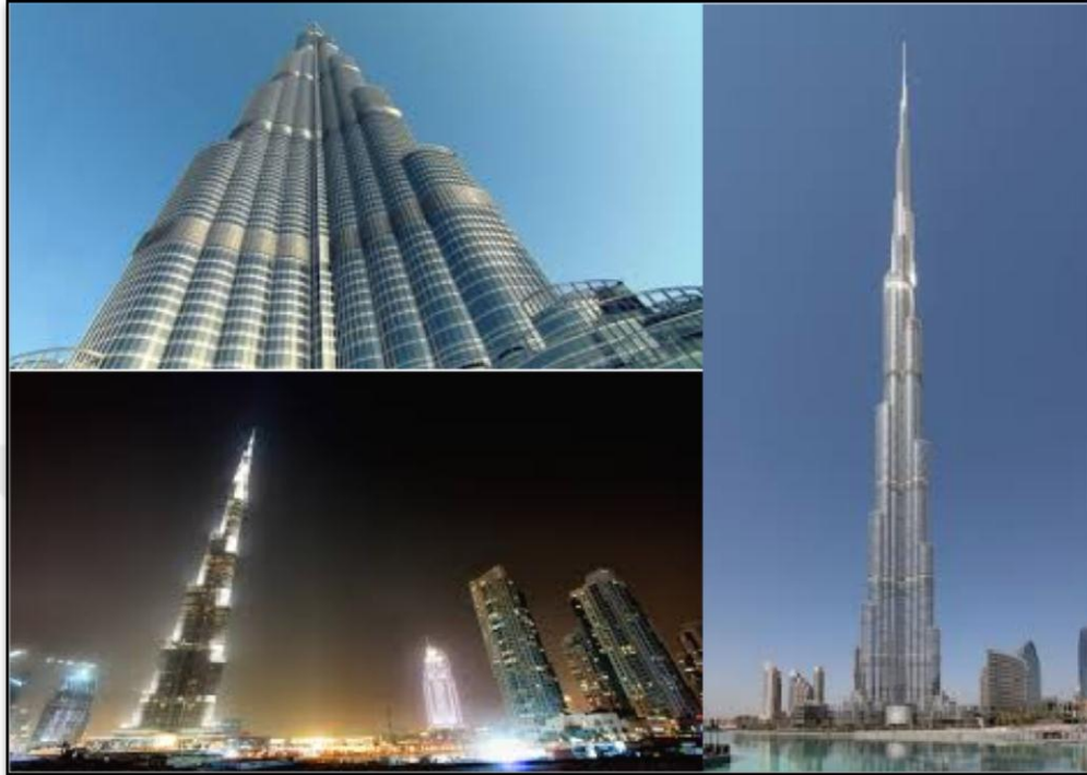
Figure 2.11 Burj Dubai tower, UAE ( http://www.burjdubai.com/ )
