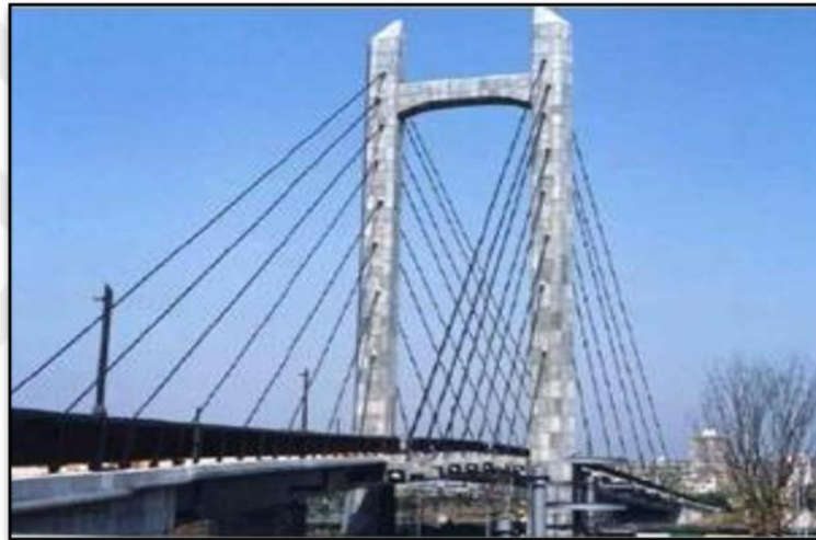
Figure 1.5 Shin-Kiba Ohashi bridge in Japan (Okamura and Ouchi, 2003)
