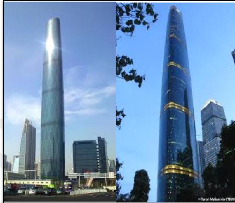
Figure 2.10 West tower project in Guangzhou, China (Feng et al., 2010)
