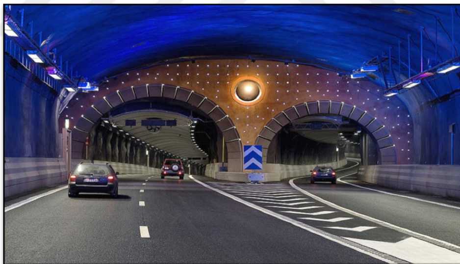
Figure 2.9 The Sodra Lanken Project (SL), Sweden (Ouchi et al., 2003)
