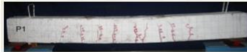
Figure 2.6 Crack pattern beam under flexure
