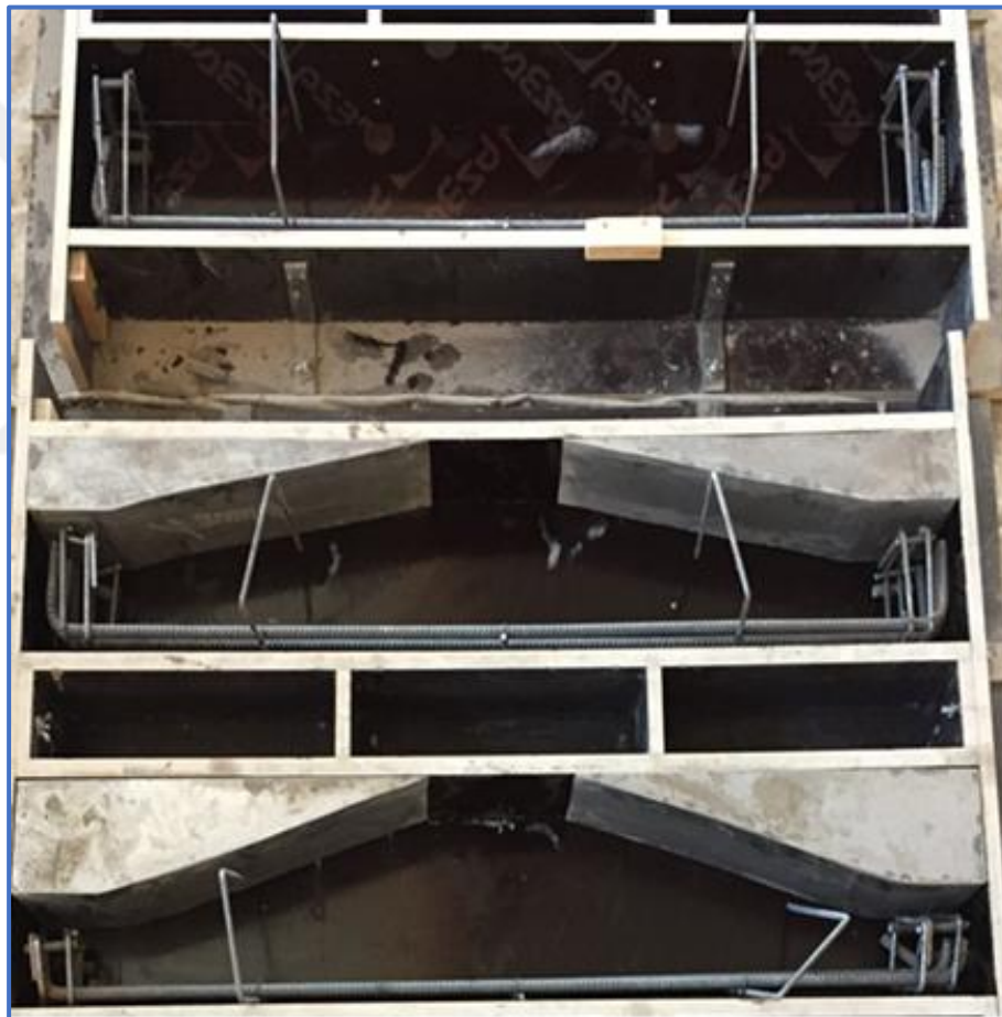
Figure 3.7 Formwork and Reinforcement Configuration for Experimented Beams.
