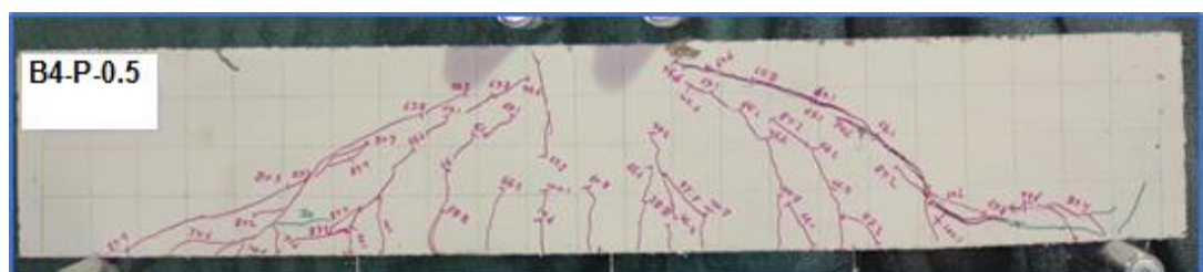
Figure 4.4 Shear Failure for Beam (B4-P-0.5)
