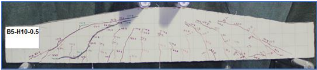
Figure 4.5 Shear Failure for Beam (B5-H10-0.5)
