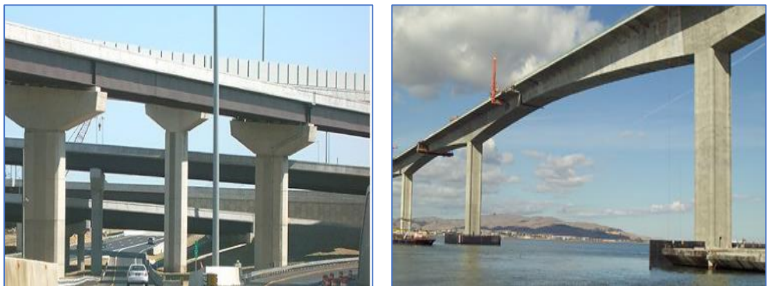
Figure 1.1 Reinforced Concrete Haunched Beams (RCHBs)
