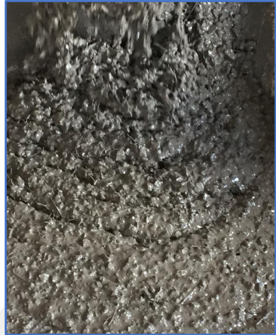
b. Steel Fiber Reinforced Concrete in Concreting Process
