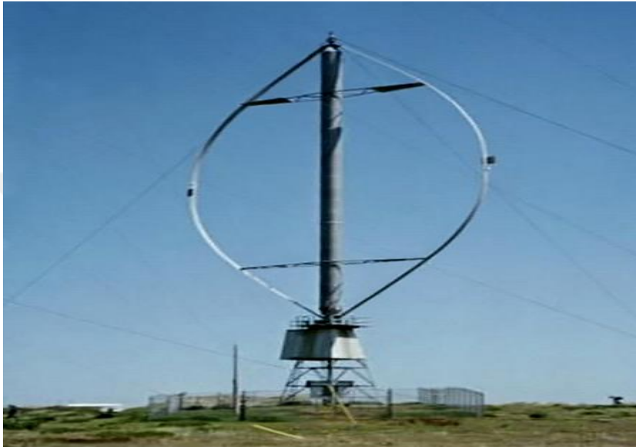
Figure 1.8 Darrieus rotor turbine
