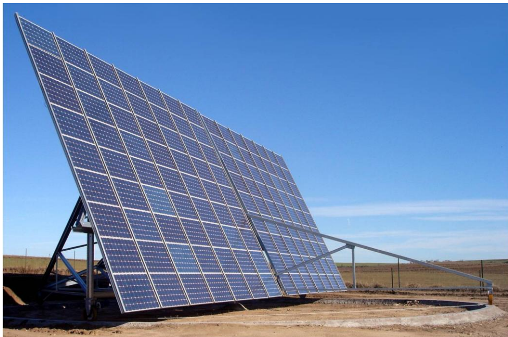
Figure 2.12 Azimuth-Altitude Dual Axis Tracker, Toledo, Spain [41]
