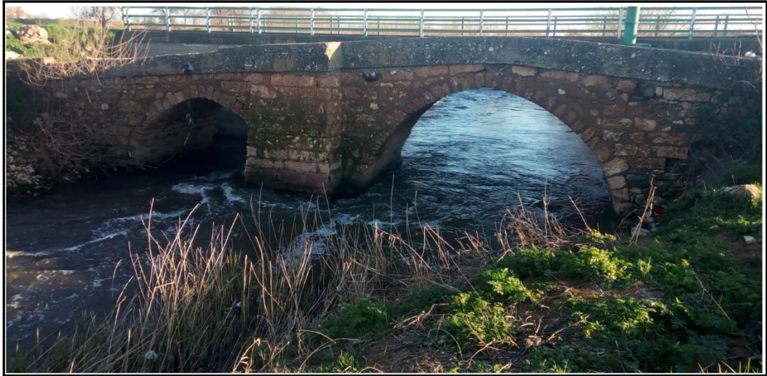
Figure 1.4 The north view of Yakacık bridge.
