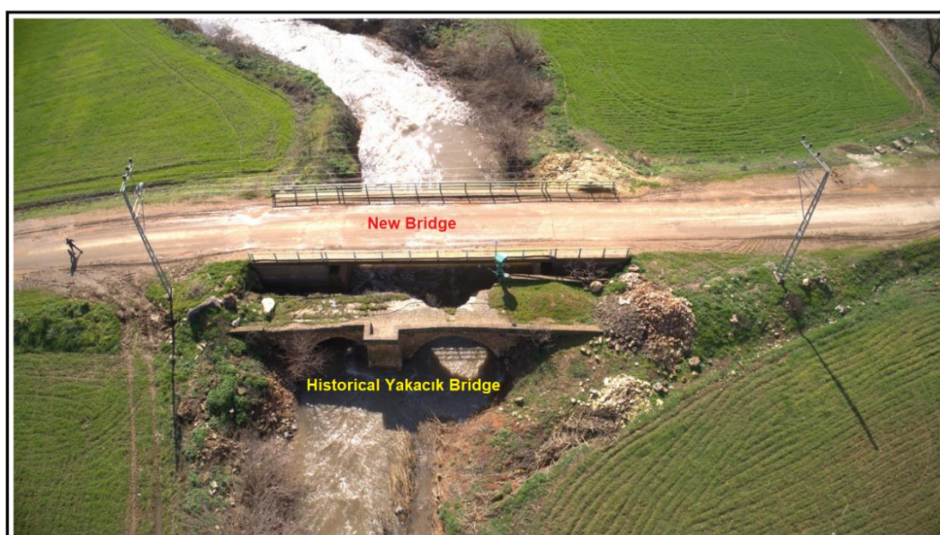
Figure 1.3 The top view of new reinforced concrete bridge and historical Yakacık bridge.
