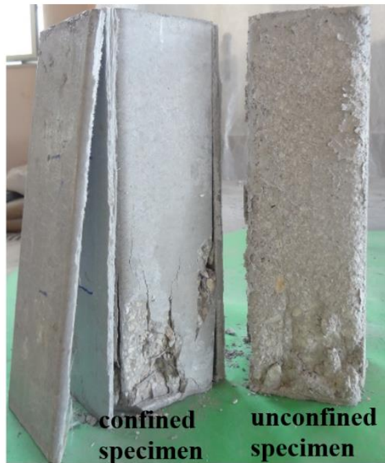
Figure 2.4 Surface degradation after acid exposure
