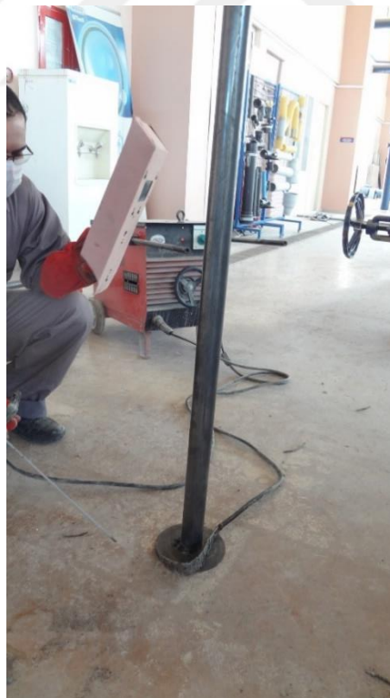
Figure (C2) prepare the inner steel tubes
