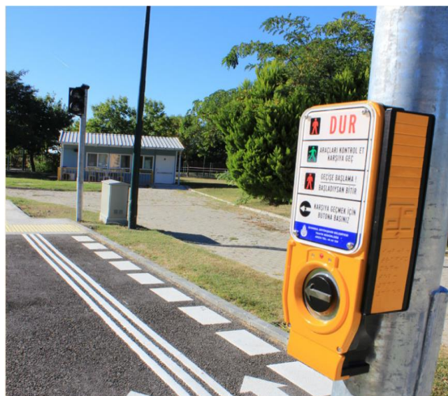
Figure 2.6 Audio orientation devices for blind
