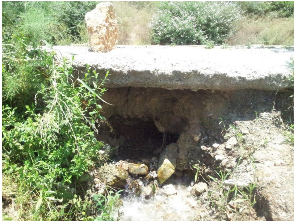
Figure 2.37. Spring discharge point 12.
