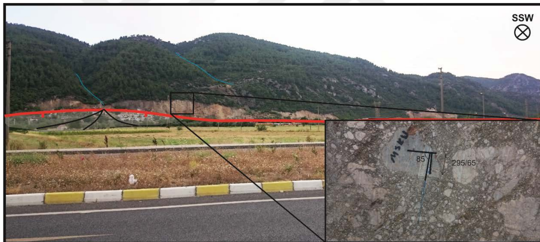
Figure 4. 18. Schematic illustration of the Paşapınarı part of Yatağan fault. SW margin of the basin is bounded by faults and resulted in the formation of hanging valleys and alluvial fan deposits. No deformation has been observed on the colluvium and alluvial fan deposits at this region.
