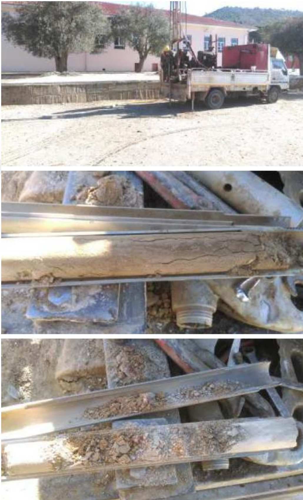
Figure A.2. Drilling Works and Their Samples for Education Building-B
