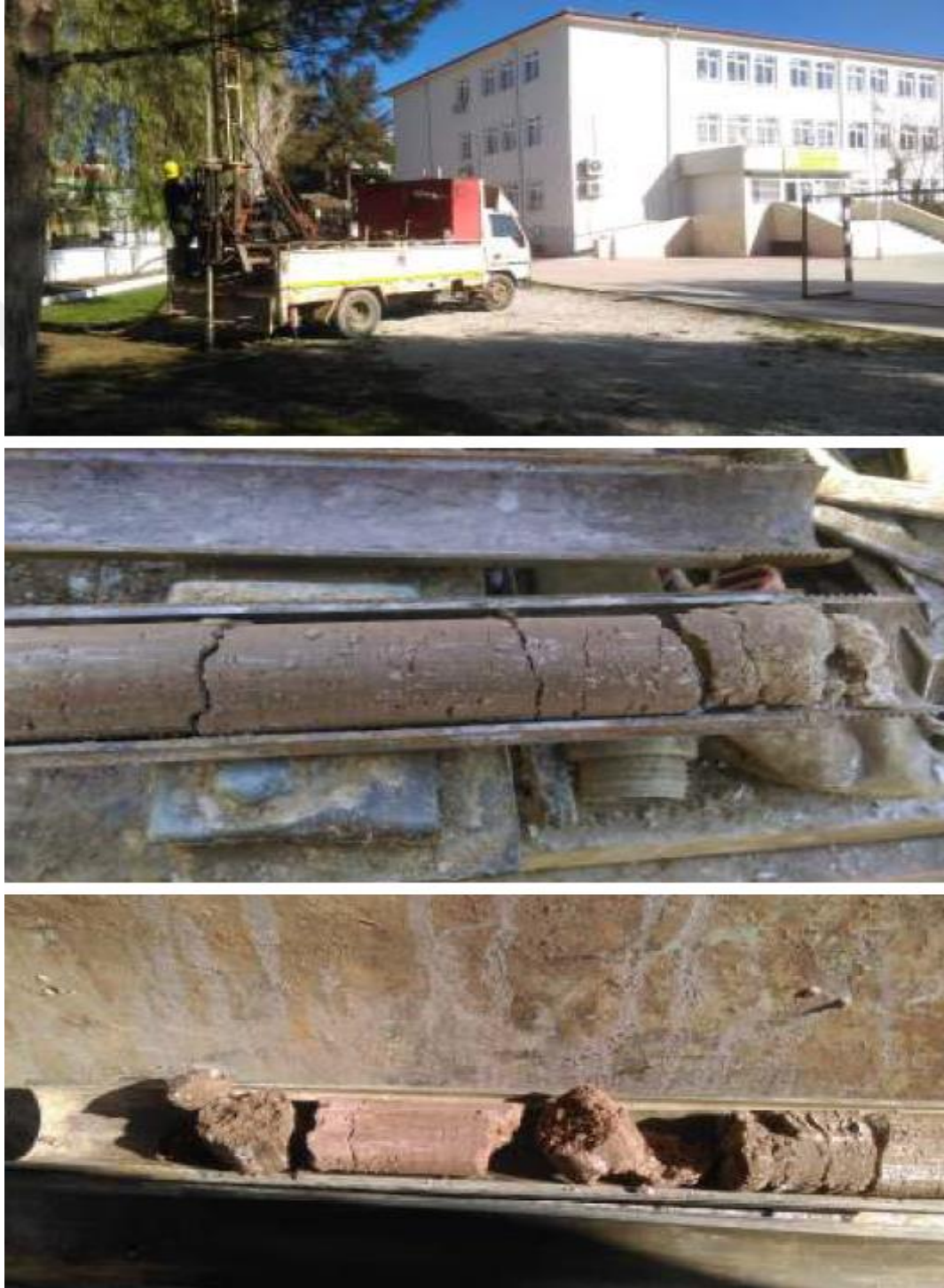
Figure A.1. Drilling Works and Their Samples for Education Building-A
