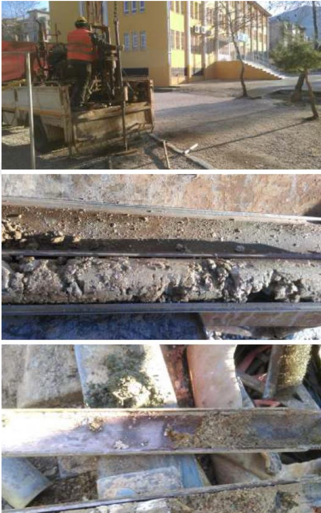
Figure A.3. Drilling Works and Their Samples for Education Building-C
