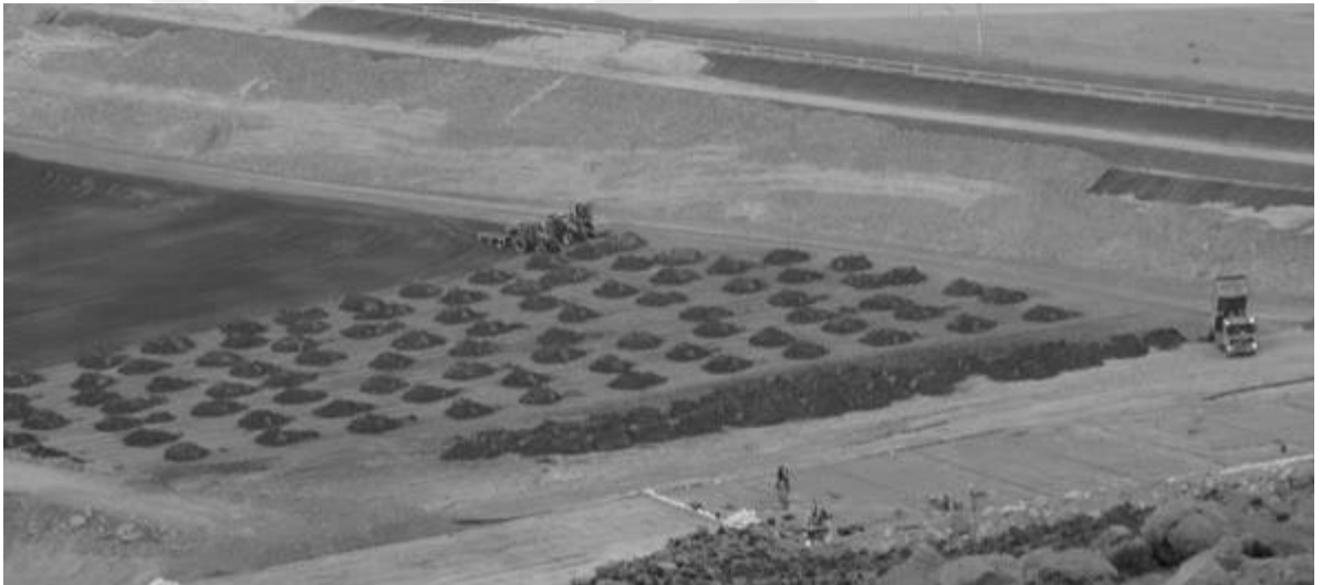
Figure 1.18. Laying Process by Truck
