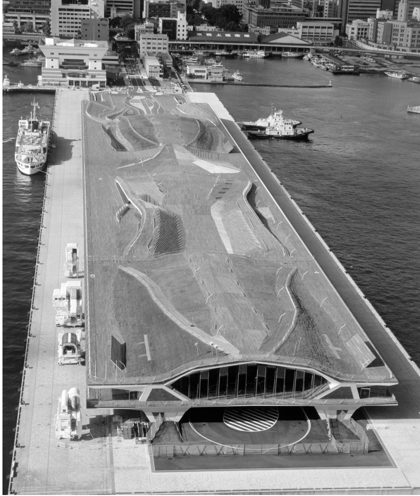
Şekil 3.9. Yokohama Feribot Terminali, Foreign Office Architects.
