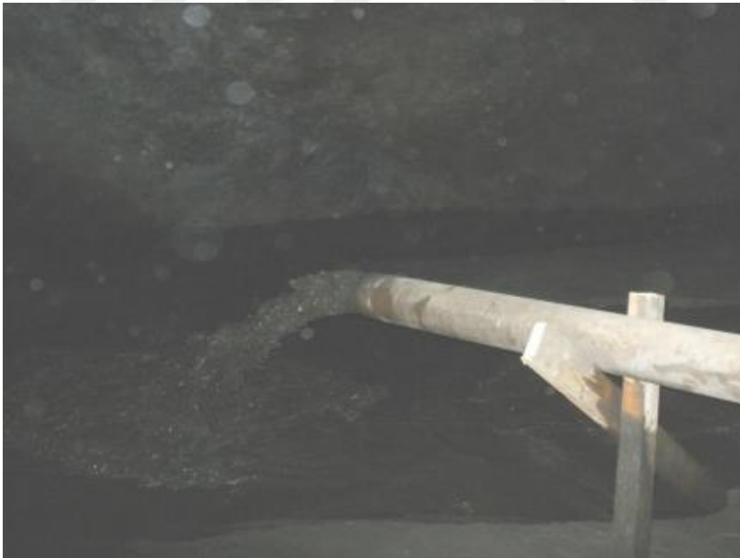
Figure 3.8. Hydraulic backfilling being poured in the mined-out stope at TUM
