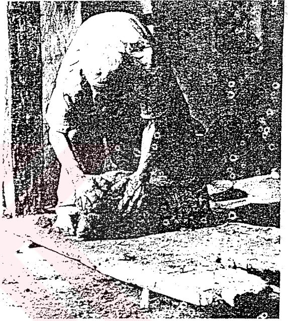
Fig. 61 Person preparing clay by adding temper and kneading it.
