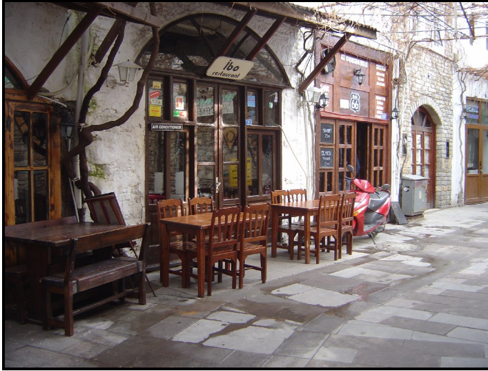
Figure 7. Window-door opening types of a restaurant in Meyhaneler Road (Photo taken by Burcu Bilgenoğlu, 2005)
